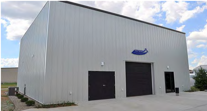
The new restoration building was completed in the spring.
